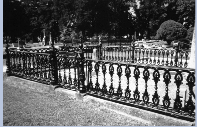
Oak Grove Cemetery's restoration effort included repairing and reconstructing iron fences surrounding many plots in the property's historic grounds, which encompasses roughly 1/3 of the entire cemetery. Using metal detectors, volunteers unearthed fence pieces as small as two inches, then numbered and put the fences back together.
